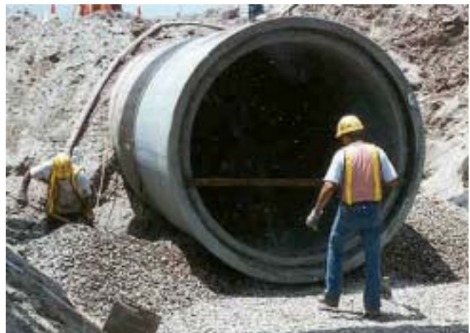
Sewer interceptor under construction
