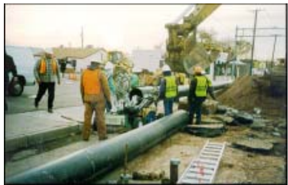
Sewer repair on Rio Grande
