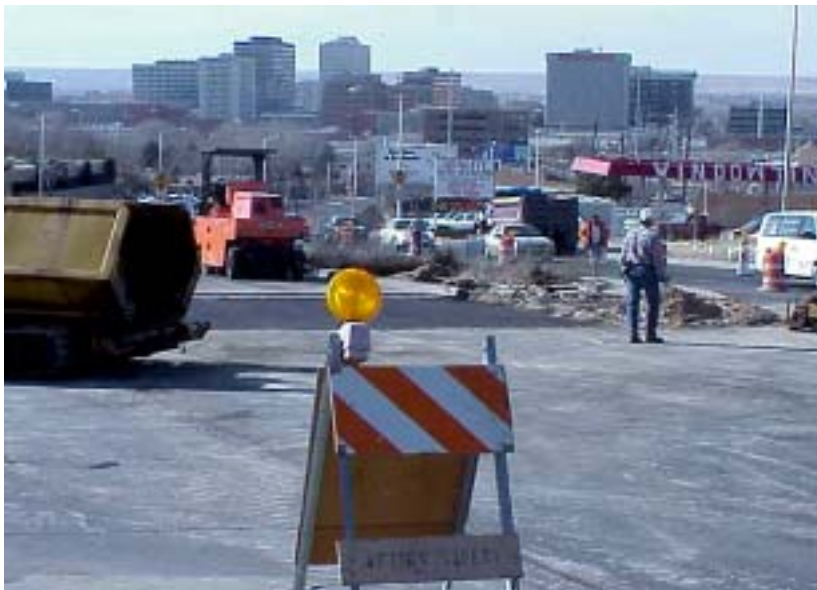
Road construction on Lomas Boulevard
