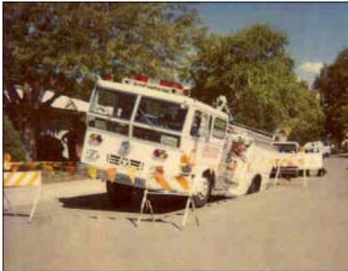
Street cave in at sewer rehab project.
