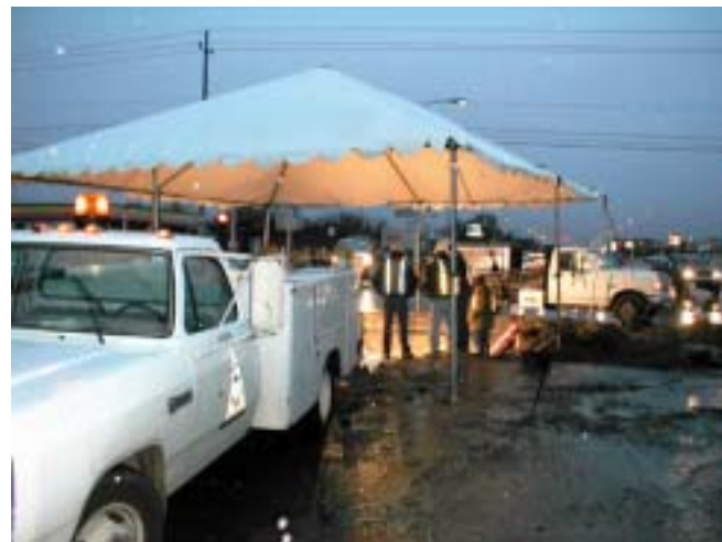
Water repair work on San Mateo
