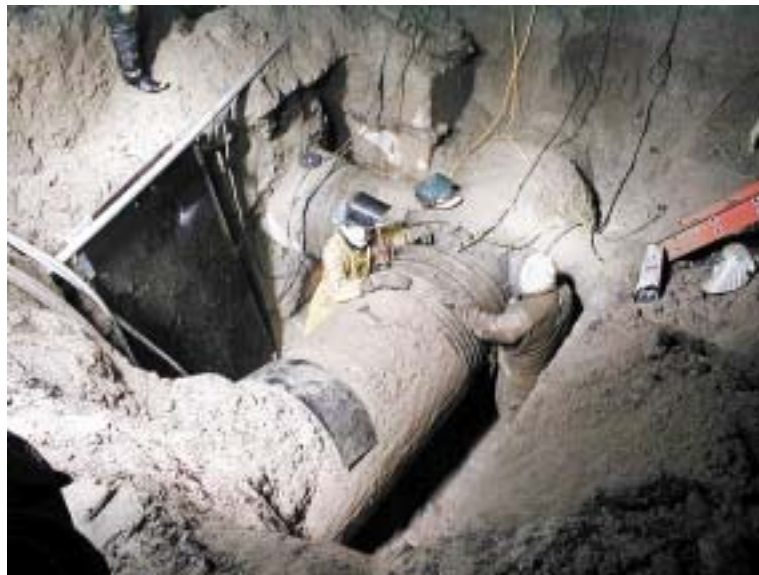
Water line rehab project
