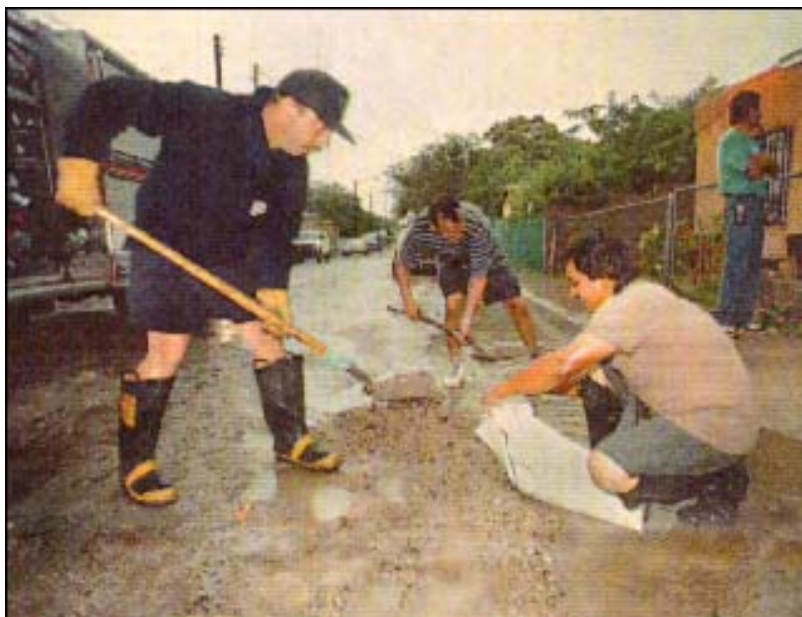
A consequence of drainage related problems
