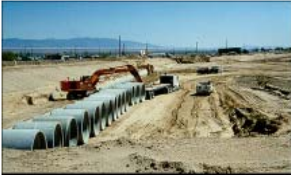
Drainage development project
